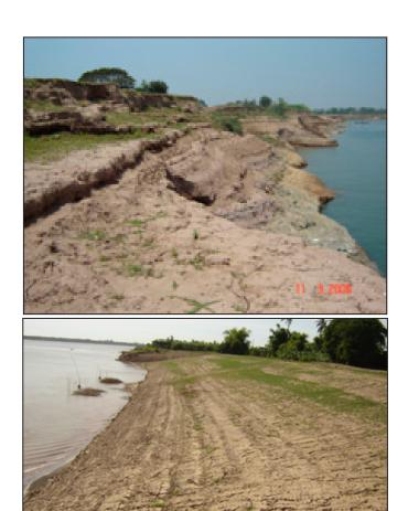
Photo 16: Eroded bank before (upper) and after earthwork (lower).
