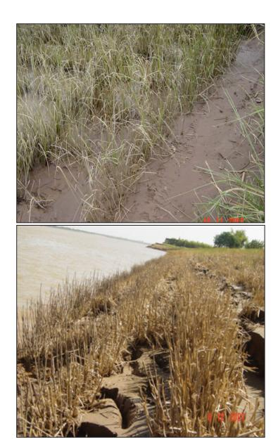
Photo 20: Upper and lower: alluvial silt deposit between vetiver rows on lower part of the slope.
