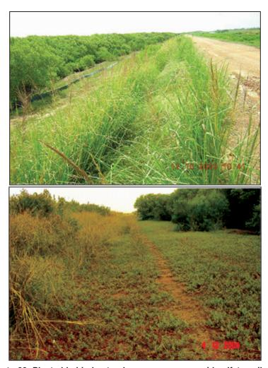
Photo 23: Planted behind natural mangrove on an acid sulfate soil sea dike in Go Cong province, vetiver reduces surface erosion and fosters the re-establishment of local grasses.
