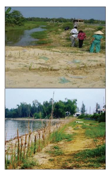
Photo 9: Upper: March 2002: VS trial at the edge of a shrimp pond, where a canal drains flood water to Vinh Dien River; lower: November 2002: mass planting combined with rock riprap to protect bank along Vinh Dien river.
