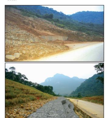
Photo 27: Da Deo Pass, Quang Binh: Upper: Vegetation cover is destroyed, revealing ugly and continuous failures of cut slopes; lower: Vetiver rows on top of the slope very slowly squeeze down, considerably reducing the failed mass.
